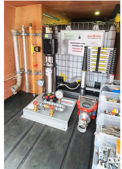
Dry Riser Test Pumps installed in customers' vans
